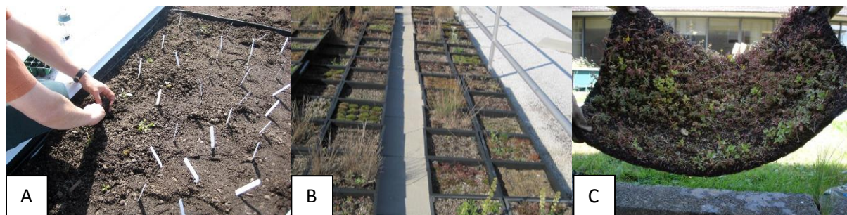
Figure 1. Examples of the three different green roof systems: A) "loose laid" system; B) modular system; C) pre-vegetated mats.
