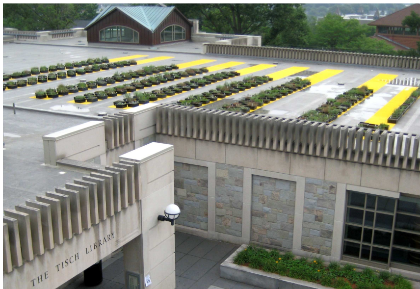
Figure 4. Experimental modular green roof on Tisch Library at Tufts University Medford, MA
