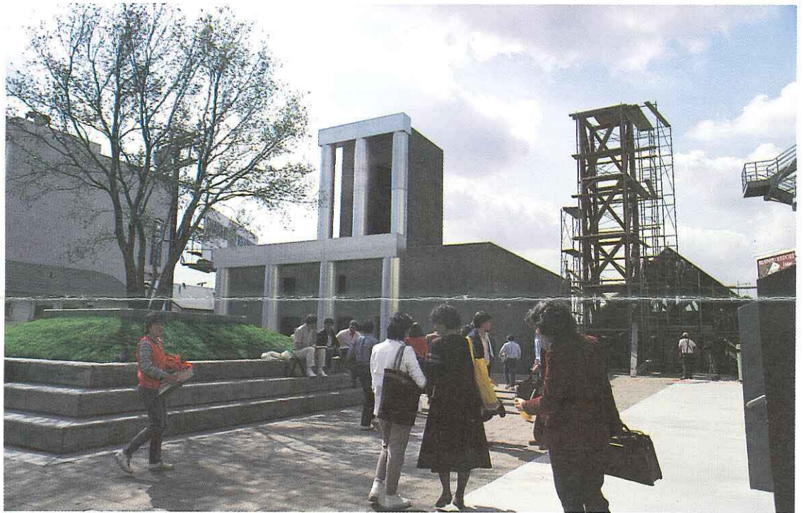
Oak Tree Quadrangle has become the campus meeting place. South Hall, a 110 seat classroom, is visible in the background and Chapel of the Advocate construction continues.
