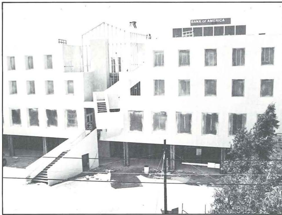
FRITZ B. BURNS BUILDING: calculated completion and occupation is for November 1981.
