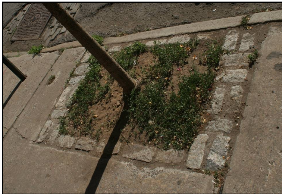
Figure 1. Typical Street Tree pit– 1.1m x 1.5m (3.5ft x 5ft).
