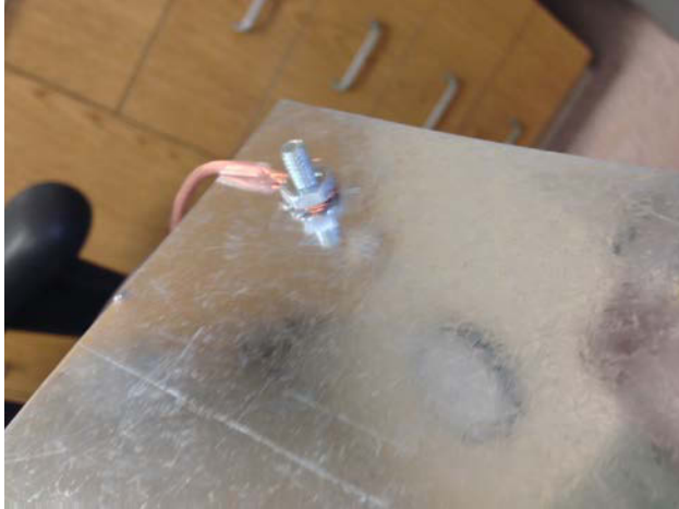
Figure 11: Bolt placed through a hole at the corner of the steel plate with a washer and speaker wire attached. The speaker wire was stripped and wrapped around the bolt with the washer tightened to secure the wires in place.
