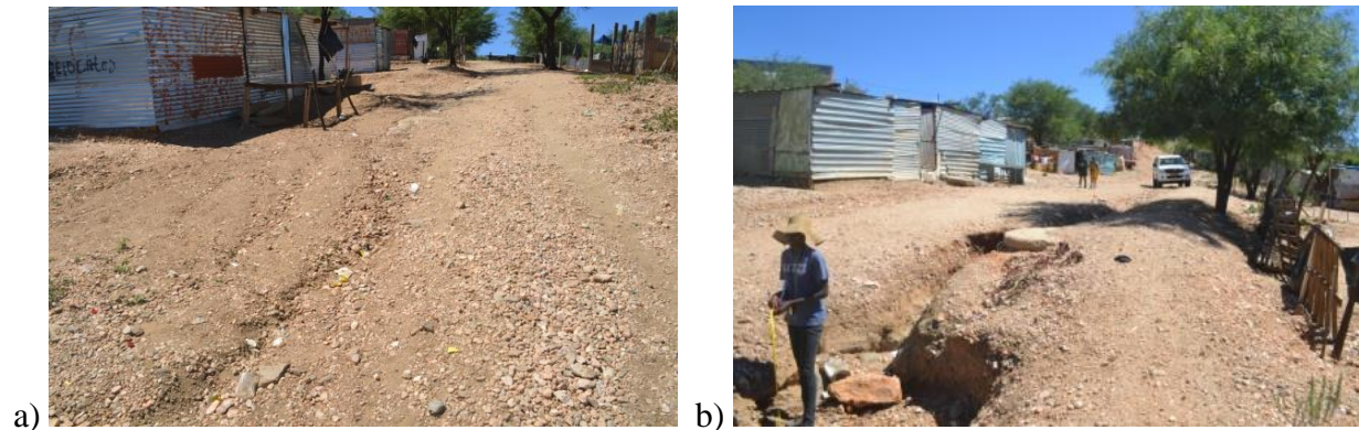
Figure 1: Photos exemplifying: (a) rills and (b) gully erosion in Okahandja Park suburb.
