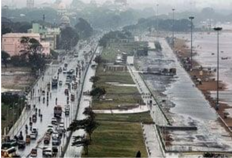
Figure 6. The Hindu, 2011. Puducherry's embankments held much of the water back, eliminating some flooding concerns.
