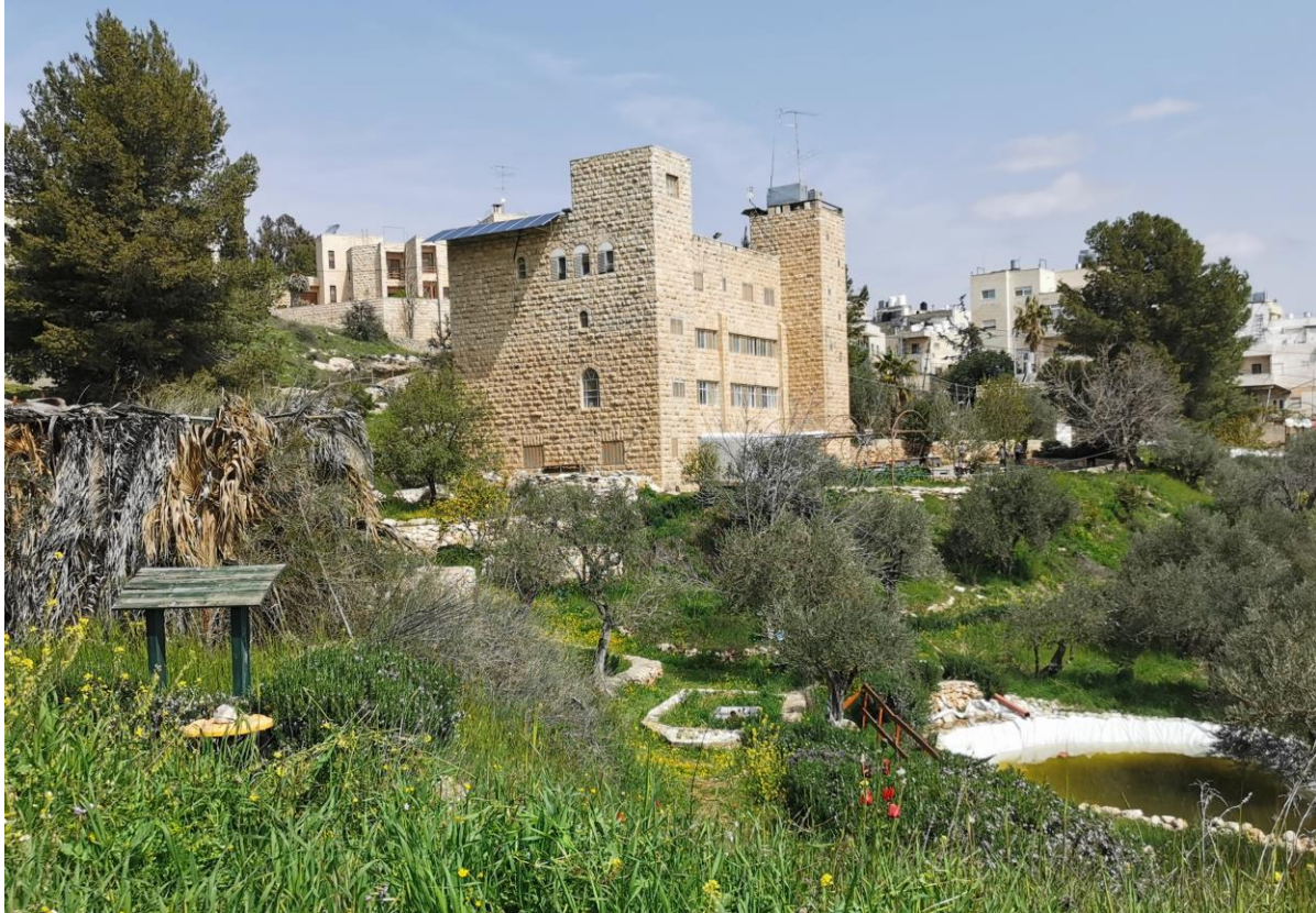
Figure 2. Rainwater harvesting pond in foreground and museum building in background.
