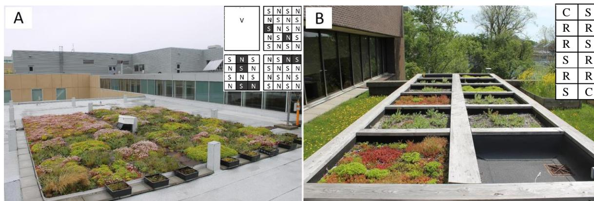
**Figure 2.** Extensive green roof at NSCC (A) and SMU (B) taken during the 2014 growing season. For the NSCC green roof only highlighted panels where analyzed. For the SMU green roof all panels were analyzed. A vegetation key is provided for both roofs: N = Native, S = *Sedum*, V = Vitaroof green roof display, R = *R. rosea* and C = Conventional roof.
